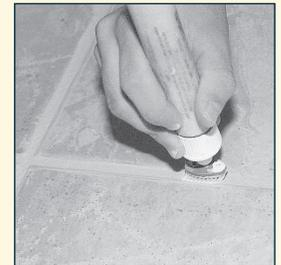
▲ Turbo Stick grout sealing tool
